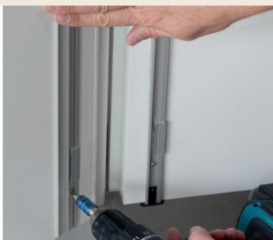
* 1. Building phase – only fixing profiles mounted
